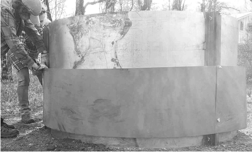
It is easiest to attach the bottom Heat Shield sheets first.
